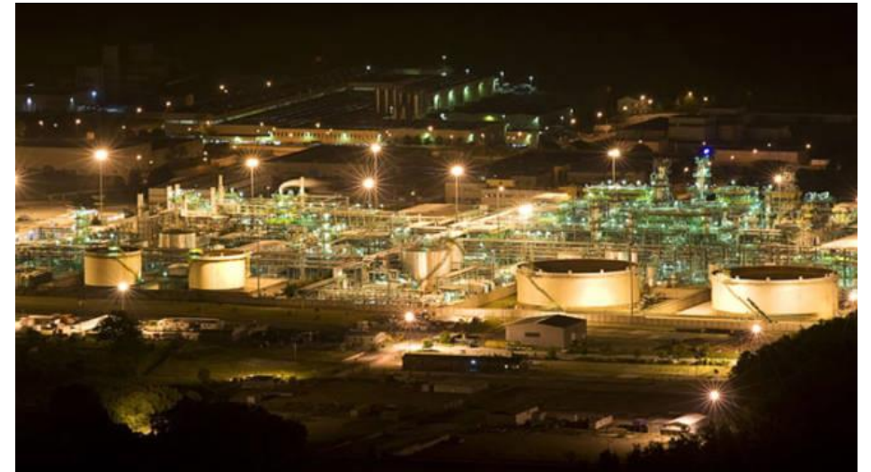
OIL EXTRACTION SITE IN VIGGIANO
